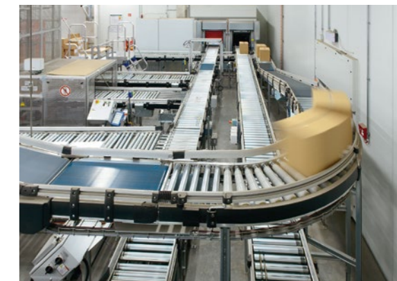
The automated small parts warehouse and the conveyor connection to the order picking area are designed for a plurality of different container sizes and qualities.
