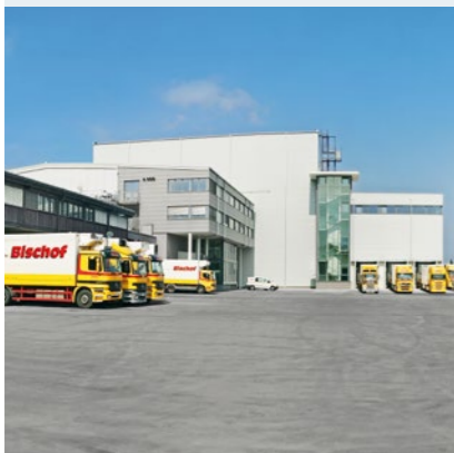
The head office in Feldkirch is the central point of a region-wide refrigerated network.
