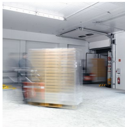
The pre-zone of the high-bay warehouse forms the interface between the manual truck loading docks and the automated storage and retrieval routes.
