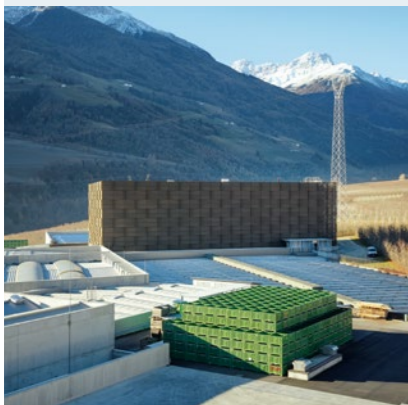
The new high-bay warehouse serves as a buffer between CA cells, sorting, and packaging.
