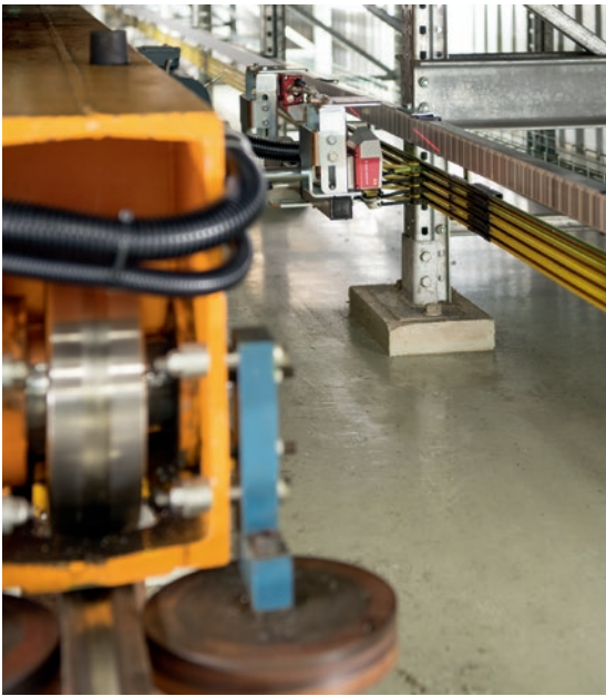
PLUG & PLAY 1: While the existing bus bar on the left side of the rack aisle remains in operation, the LTW team is already installing the new bus bar including bar code distance measurement on the right side. All that needs to be done on the agreed date is to switch them over.
