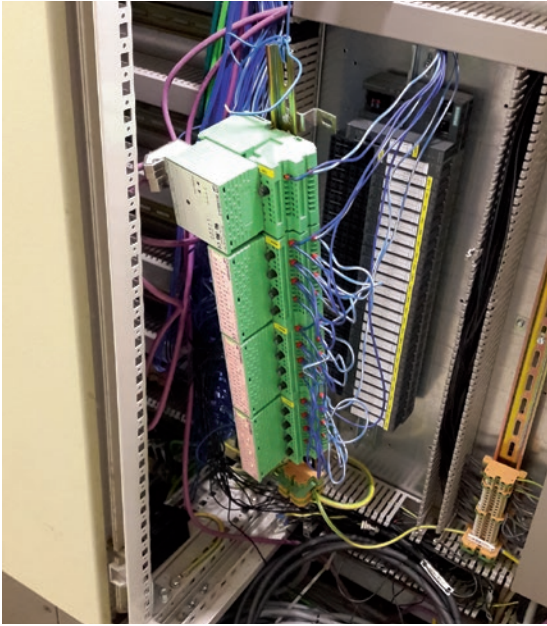
PLUG & PLAY 2: Pre-installation of the new control during operation of the old components that have already been partially taken out of the control cabinet.
