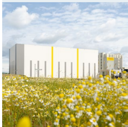
With a cubage of 72,000 m 3 , one of the biggest wooden high-bay warehouses in the world.
